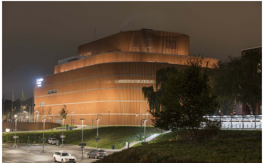
Exergi Power Station, Stockholm. Architecture: Urban design, Stockholm. Photography: Johan Elm, Stockholm.
