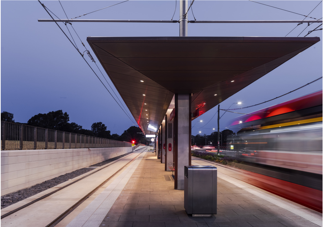
Sydney Light Rail, Sydney. Architectuur: Grimshaw. Lichtplanning: Electrolight, Sydney. Fotografie: Jackie Chan, Sydney.
