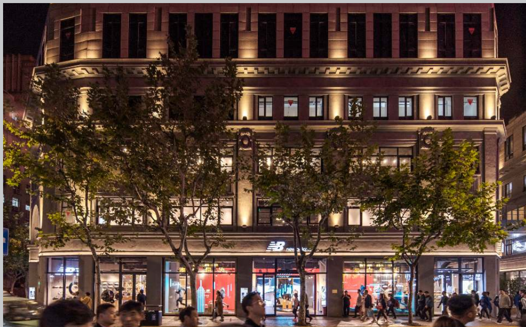
The Central Mall, Shanghai. Archi- tektur: East Chi- na Architectural Design Institute, Shanghai Zhang Ming Architectu- ral Design Institu- te & CallisonRTKL. Lichtplanung: Shanghai New Century Lighting Co., Ltd. Fotogra- fie: Jackie Chan, Sydney.
