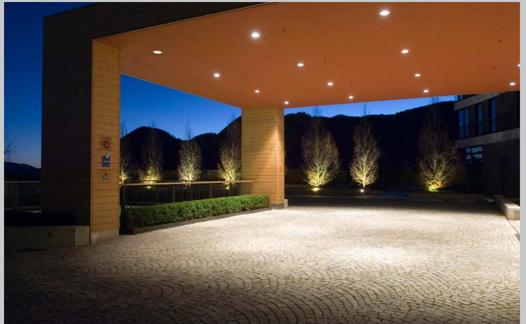
Intercontinental Resort, Berchtes- gaden. Architect: Kochta Architek- ten, Munich. Elec- trical design: Ingenieurbüro Schnell, Tuttlin- gen.
